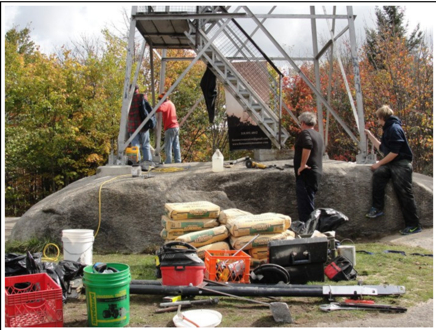
Construction site near the completion of the job.
