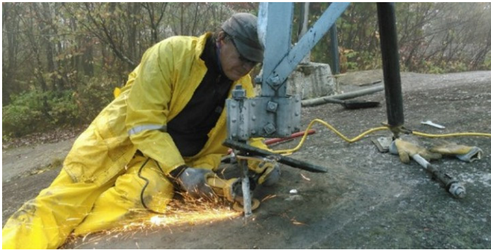
How does a fire tower put its new footers on?... One leg at a time, just like everybody else
